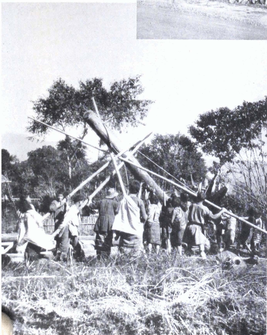
16. Building a Kachin house; lifting the main post
